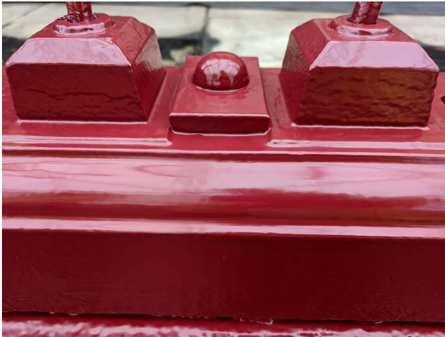
Plinth of parapet with top coat
