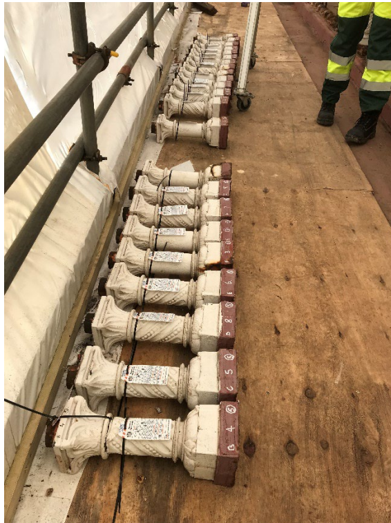
Balusters removed awaiting refurbishment
