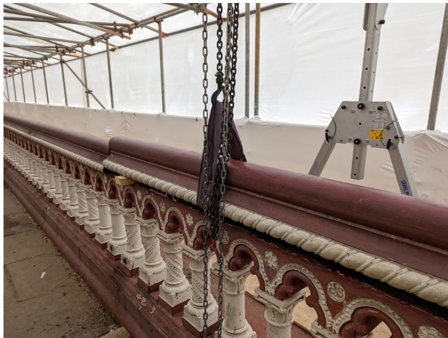
Top Rail being removed
