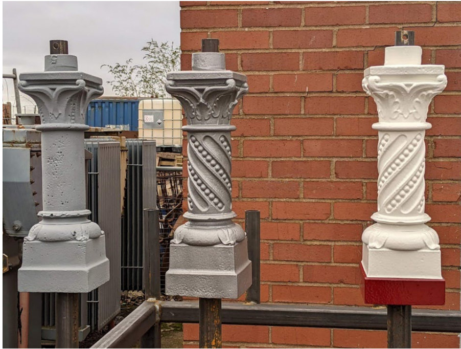
Refurbished balusters; Primed, undercoated, top coat (Wolverhampton)
